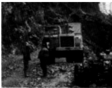
Road construction through tough terrain in May, 1983
