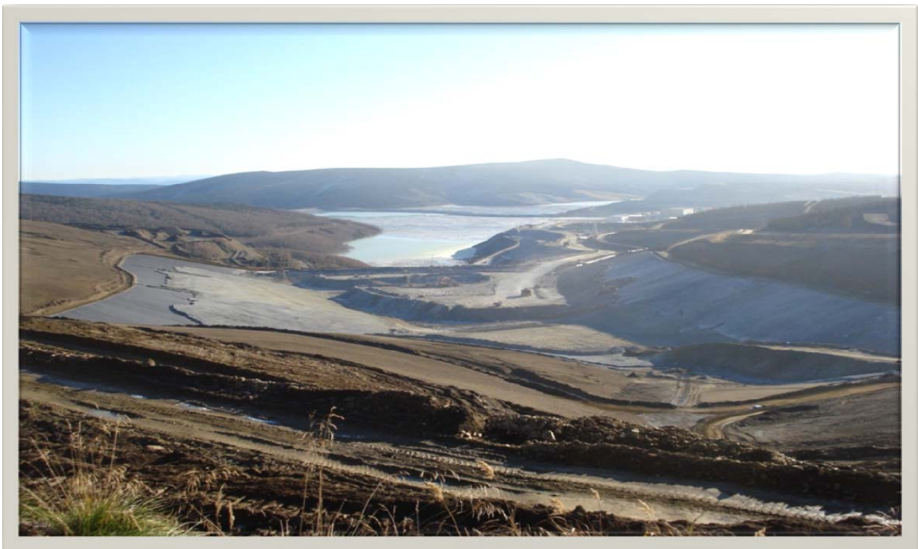
Walter Creek Valley Heap Leach – October 14, 2009
