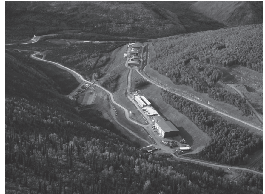
Aerial view of plant site at Pogo Mine (Teck Cominco 2007a).
